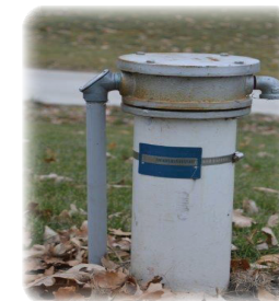
Well in good condition
